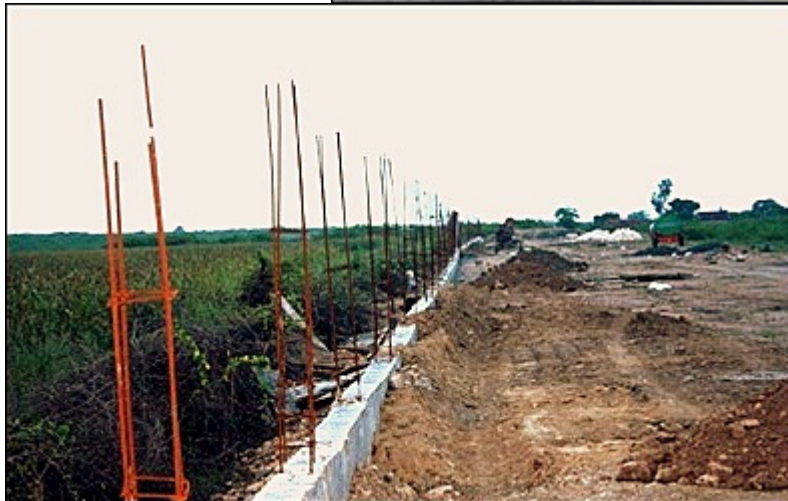
Boundary wall along IMC Plot
