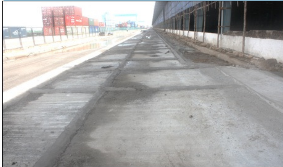
Road between Fertilizer Shed & RMGC Yard
