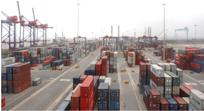
Container Yard Works- Complete & in use
