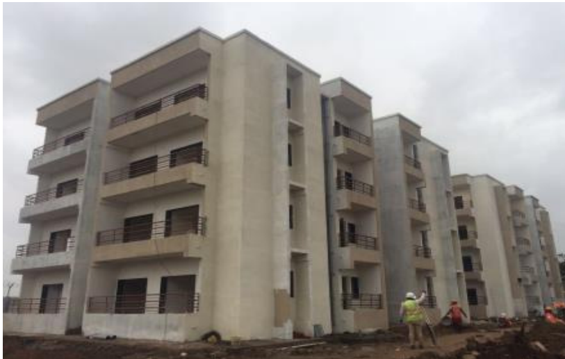
Construction of Residential Building
