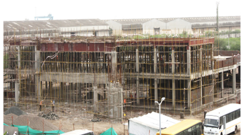
Construction of Office Building Commenced
