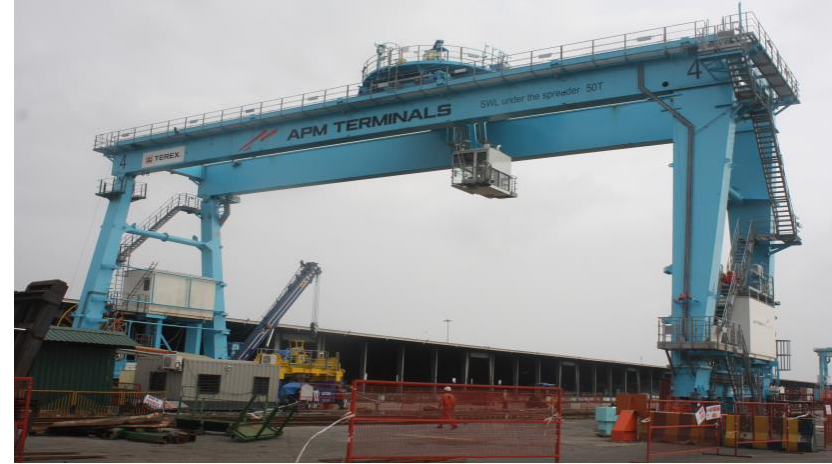
RMGC- Expected completion August 2016
