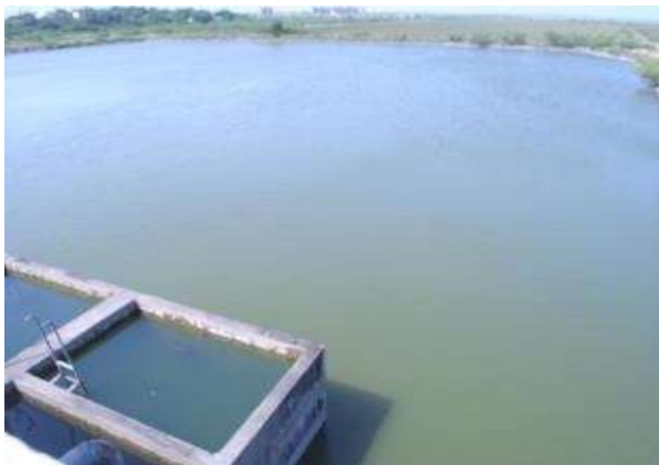
Dust Suppression Water Reservoir
