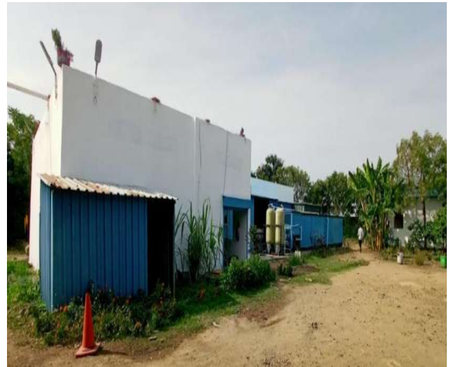
450 KLD STP for Residential Area
