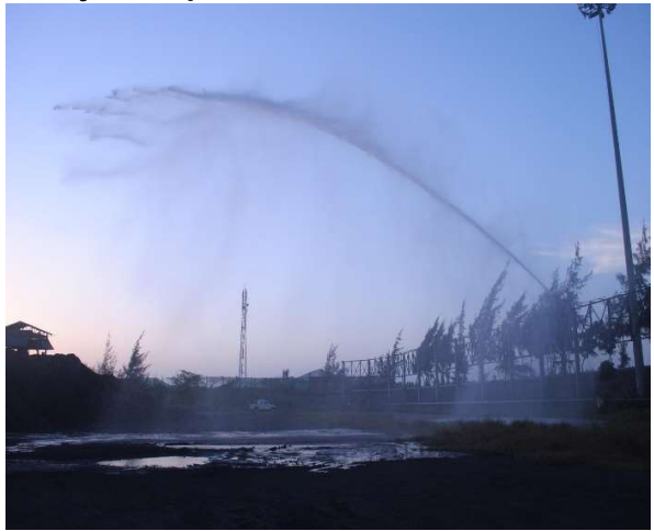
Water Sprinkler in Coal yard
