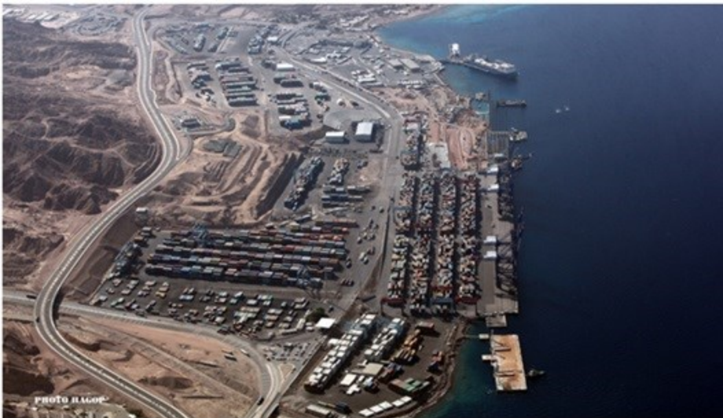
ACT - Aqaba Container Terminal (Total Surface 55 Hectares)
