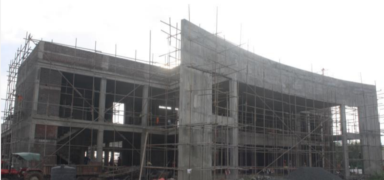
Construction of Office Building at Port
