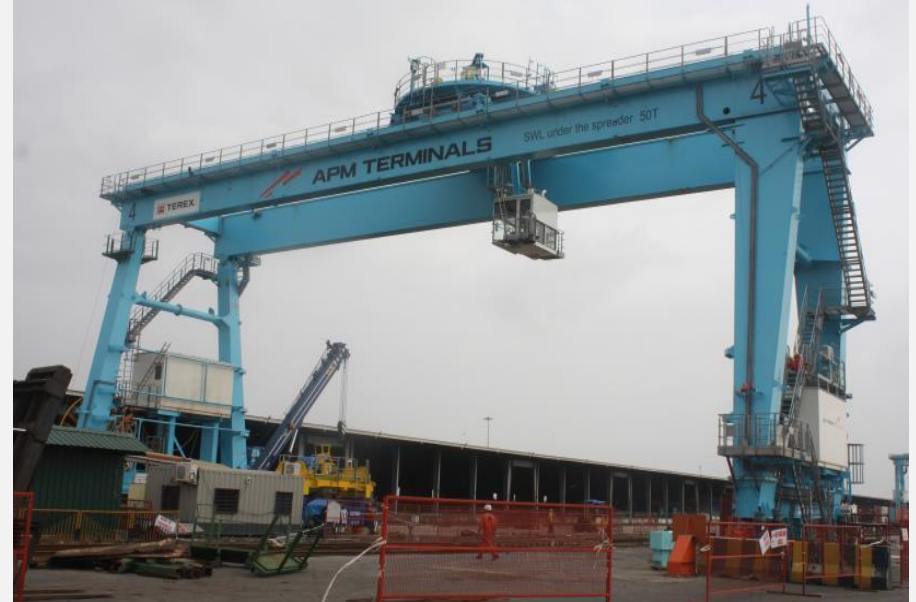
RMGC- Installation and Testing In progress.
