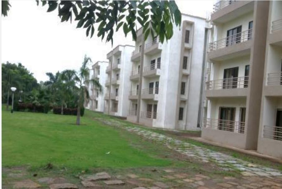
Construction of Residential Building at the Port
